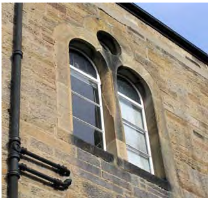
Above: stone decay (Block E)
