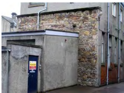
Below: fragment of the original rubble stone boundary wall to the brewery at the north end of the old clinical block
