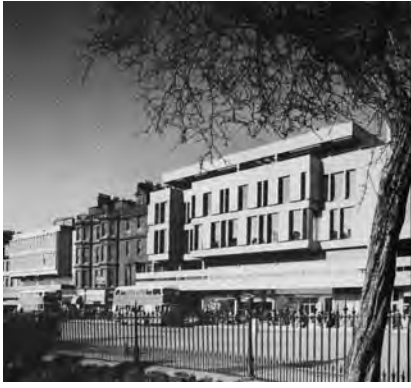
Above: contemporary photograph of the New Club, Princes Street, Edinburgh by Alan Reiach, Eric Hall & Partners when complete (1969)
