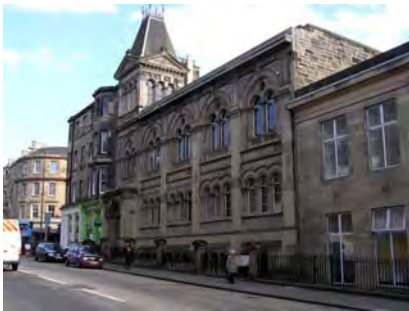
Below: former Hope Park and Buccleuch Congregational Church and details of the façade on Hope Park Terrace (1876)
