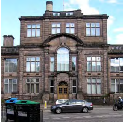
Above: the centrepiece of the façade to Summerhall
