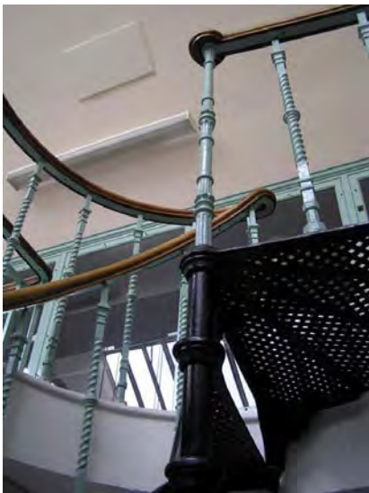
Upper: first floor corridor within the main teaching block
