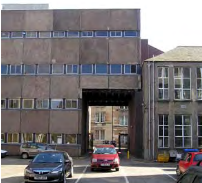
Above: rear of Block B viewed from the courtyard
