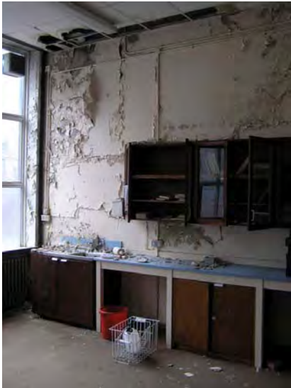
Above: decaying finishes within the former clinical department
