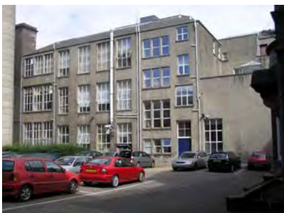
Above: rear elevations of the main teaching block
