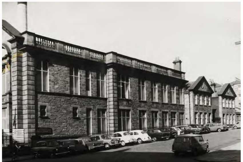
Right: photographs taken c1970 before the demolition of the pavilions at the rear of Summerhall Square, and the archway leading to the rear courtyard to accommodate Block B © EUL
