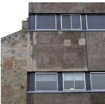
Above: concrete repairs, Block B
